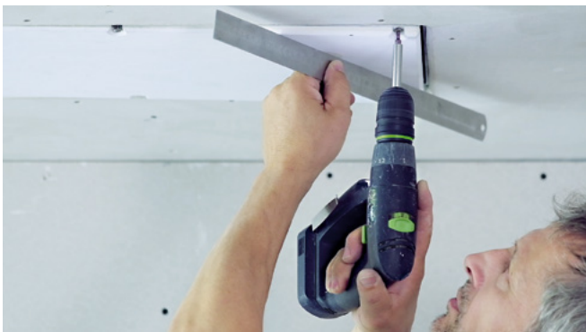
Fix all the screws and adjust the speaker so it is flush mounted. All screws must be under tension.
