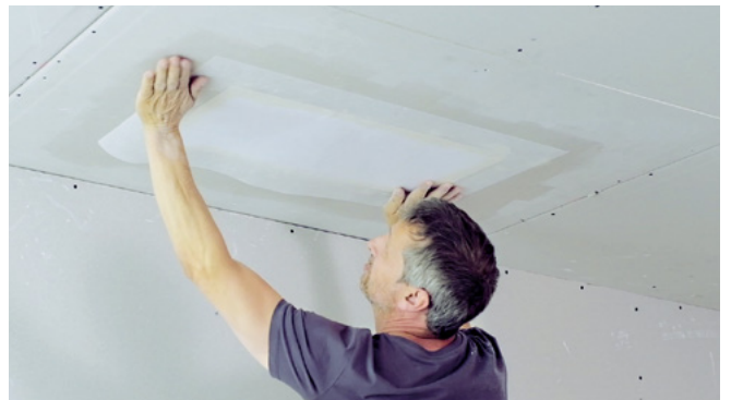
and attach the lining. Leave to dry for at least 24 hours!
