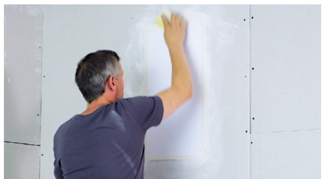
Sand the entire surface of the membrane using light pressure.
