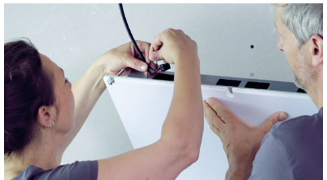
Connect the speaker cable and tighten the cable tie. Insert the speaker and attach it by fixing the first two screws.
