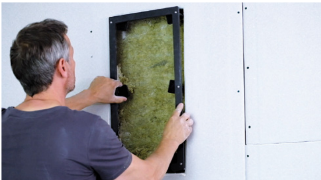
Insert the mounting feet and assembly frame...
