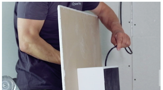
Insert the cable into the back box...
