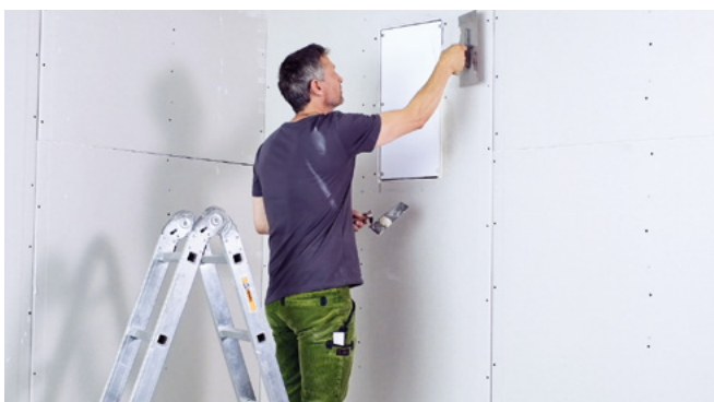
Plaster twice over the edges and drill holes. Leave to dry for at least 24 hours!
