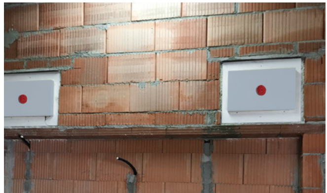
EGB Plan 400 back boxes in a solid wall
