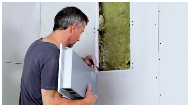
Connect the speaker. Tighten the cable tie.
