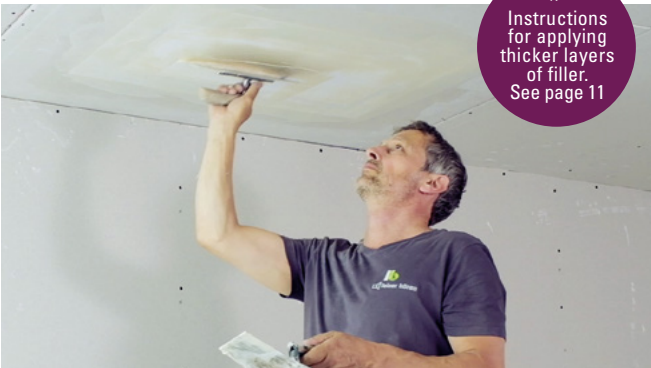
Apply 1-2 thin layers of plaster over the entire surface. Leave to dry for at least 24 hours!
