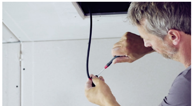
Attach the system terminal to the speaker cable. Make sure the polarity is correct.
