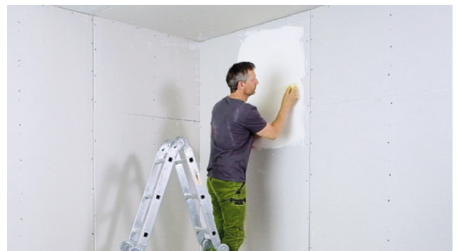
Sand the entire surface. Only apply light pressure over the membrane.
