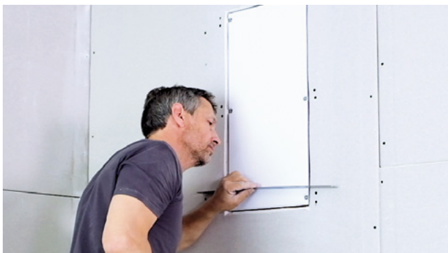
Adjust the speaker so it is flush mounted. All screws must be under tension.
