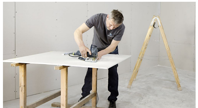
Cut the installation opening. For round openings, use a circle cutter to cut out the installation opening.
