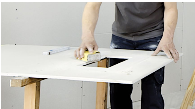
Trim the installation opening and sand the edges.
