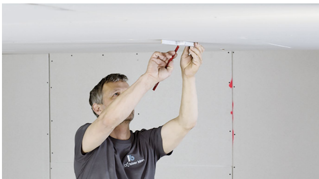
Locate and mark out the installation position.
