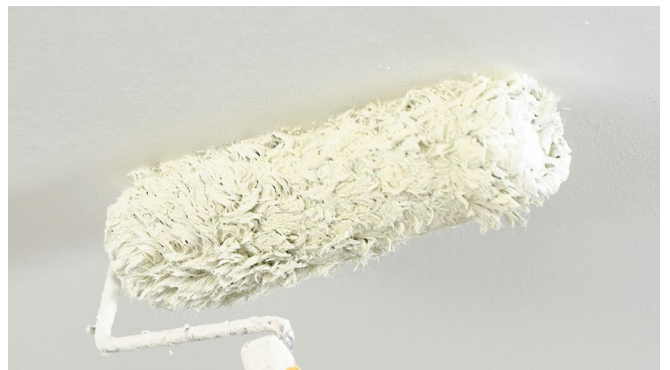
and paint the entire area.
