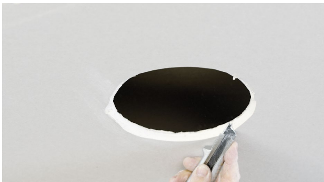
Trim the installation opening...
