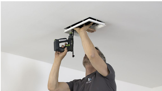
Insert frame into opening and screw in place. The springs are not used.
