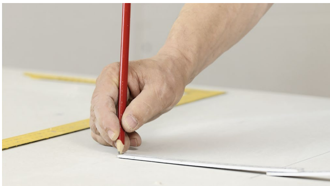
Locate and mark out the installation position.
