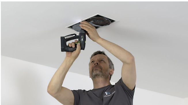
Insert speaker module and fix in place.
