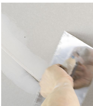
Plaster and paint.
