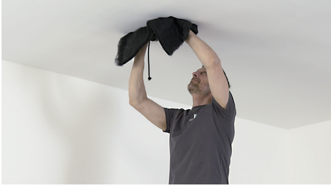
Line the box with insulating wool.
