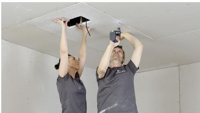
and screw the plasterboard in place.
