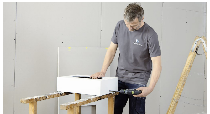
Drill a hole in the back box for the cable.
