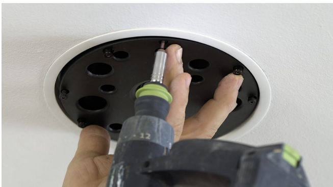
and fix in place.
