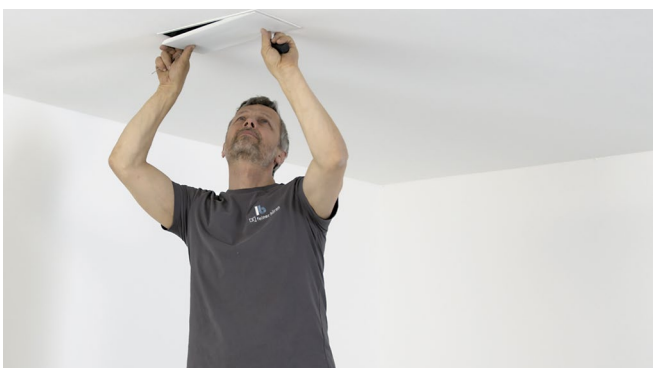
Insert the grille. Realign the fixing magnets if necessary. Revision: Remove the grille using the magnetic DE tool.
