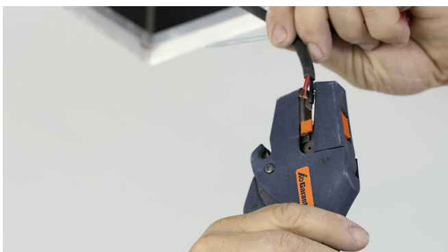
Isolate the speaker cable. Make sure the polarity is correct.
