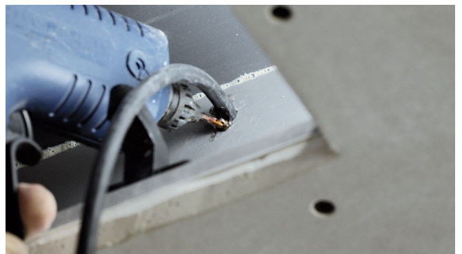
Seal the cable hole in the back box (using hot glue or sealing compound).
