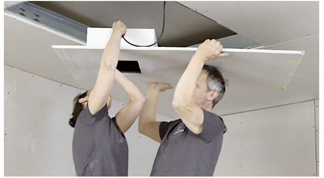
Guide the cable into the back box...
